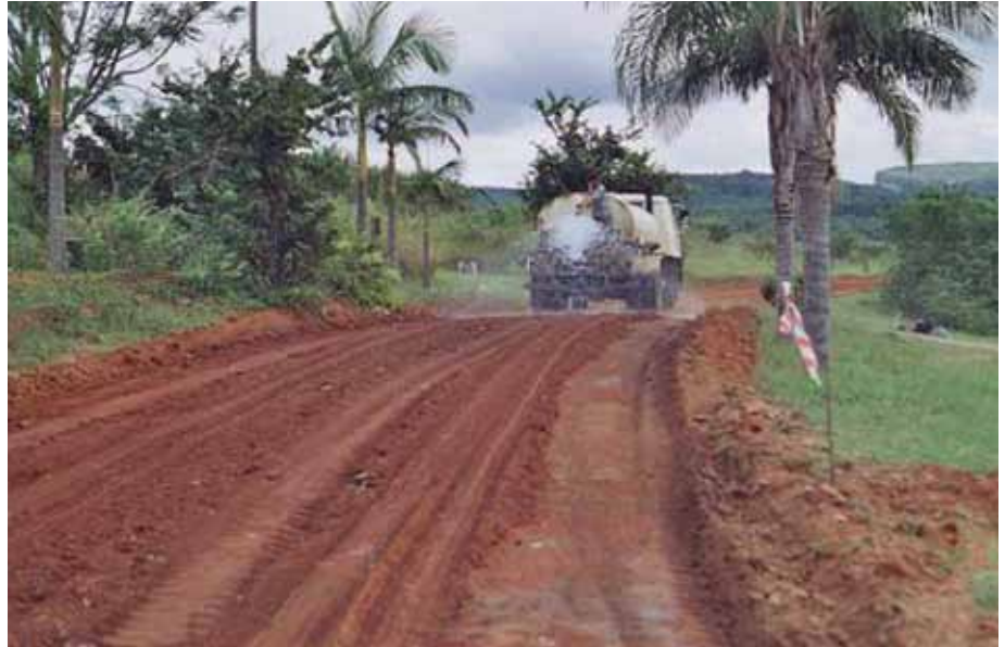
A TRUCK SPRAYS AGGREBIND ON A ROAD IN A GAME PRESERVE IN SOUTH AFRICA. AGGREBIND STRENGTHENS AND HOLDS TOGETHER RAMMED EARTH STRUCTURES, ALLOWING FOR CHEAPER CONSTRUCTION WITHOUT AGGREGATE.
