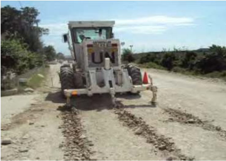
Picture 03: Initial situation and scarification.
