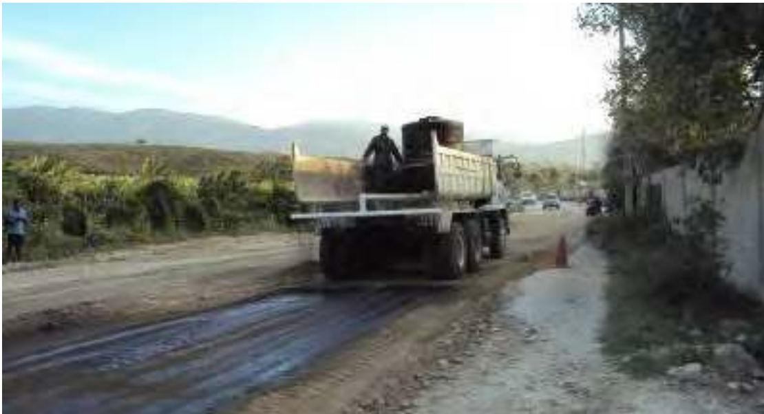
Picture 09: Application of the mixture - Aggrebind: water.
