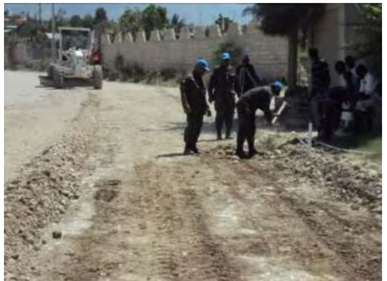
Picture 06: Repair of broken pipe.
