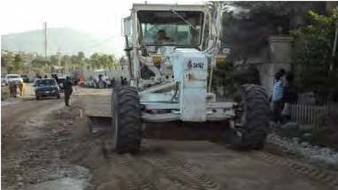
Picture 08: Ground leveling.
