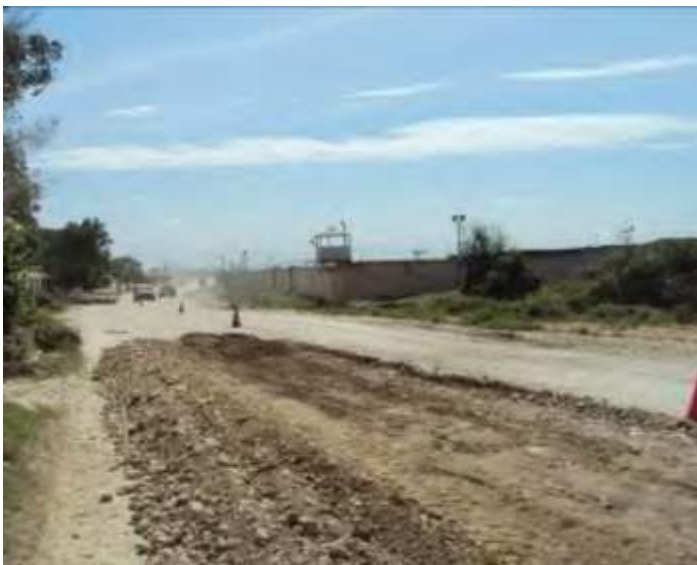
Picture 05: Cut and removal of 15 cm of natural soil.
